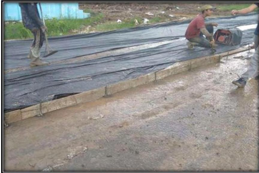
Gambar 4.5 Pemasangan *Plastic Sheet*
